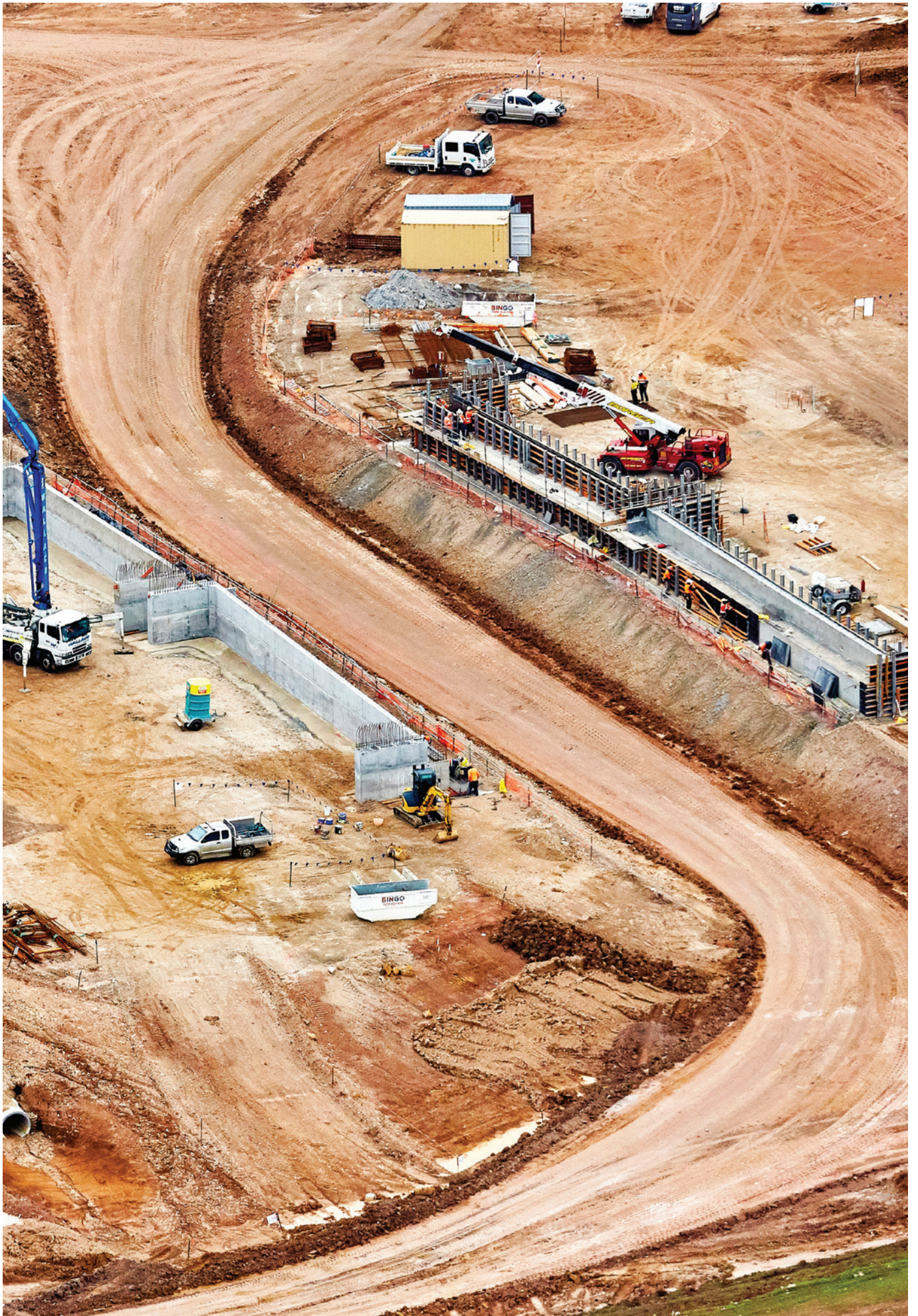
Early earthworks on-site
