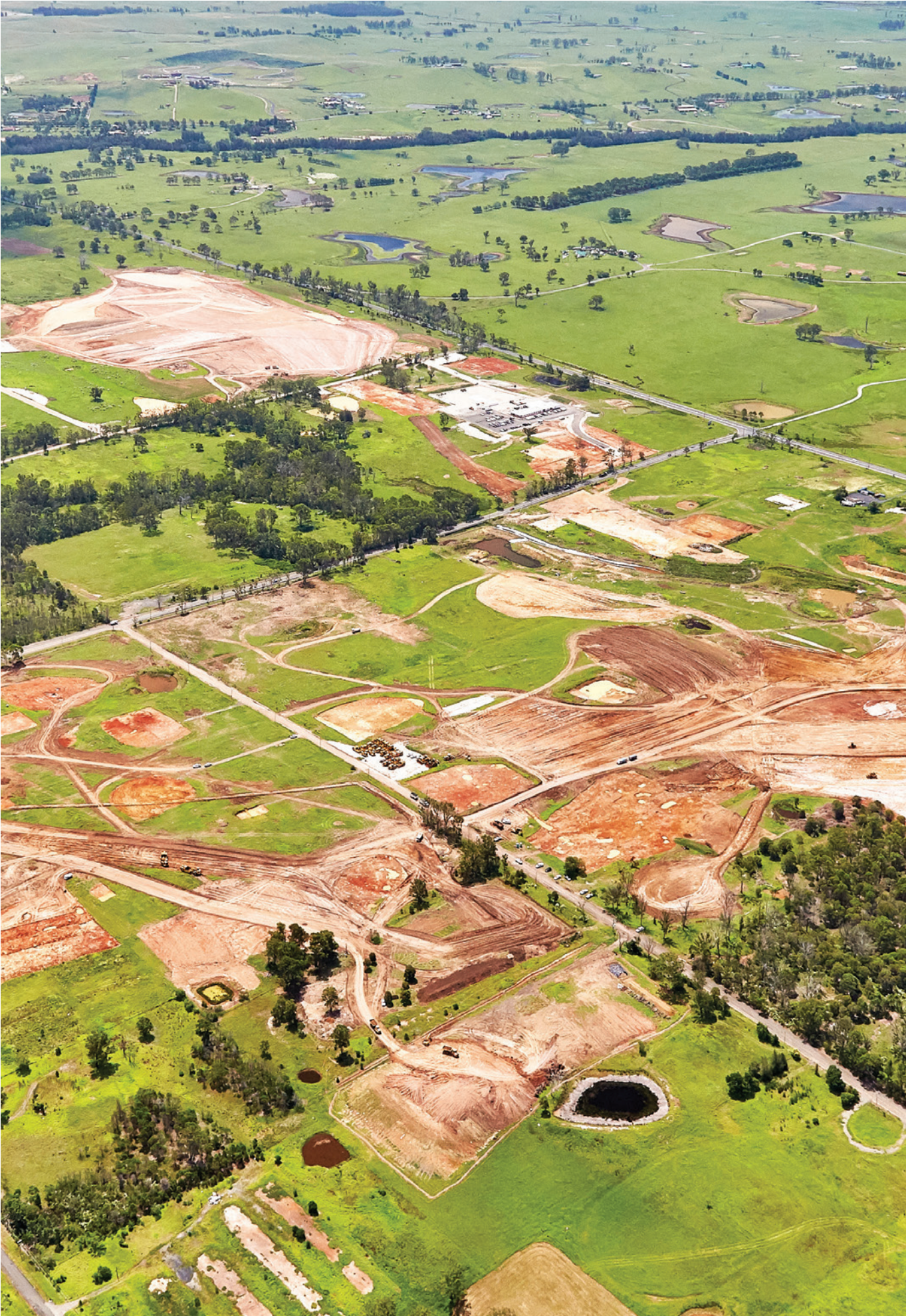
Early earthworks on-site
