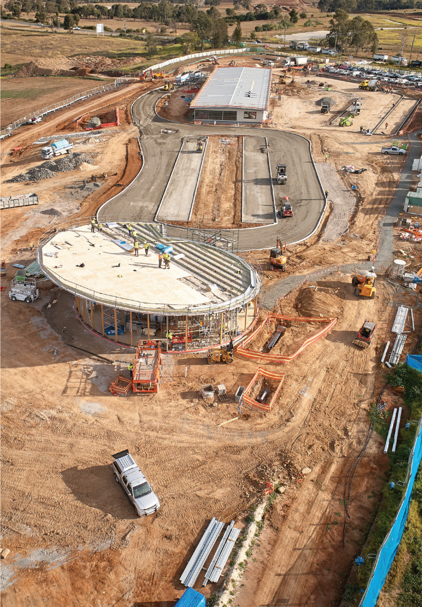
Construction of Experience Centre and Site Office.
