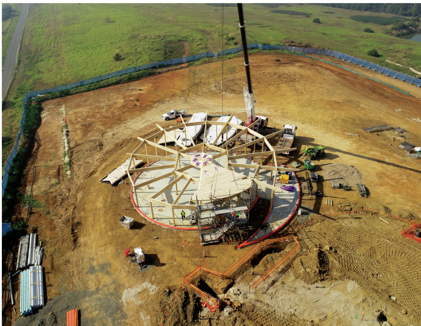
Construction of the Experience Centre.
