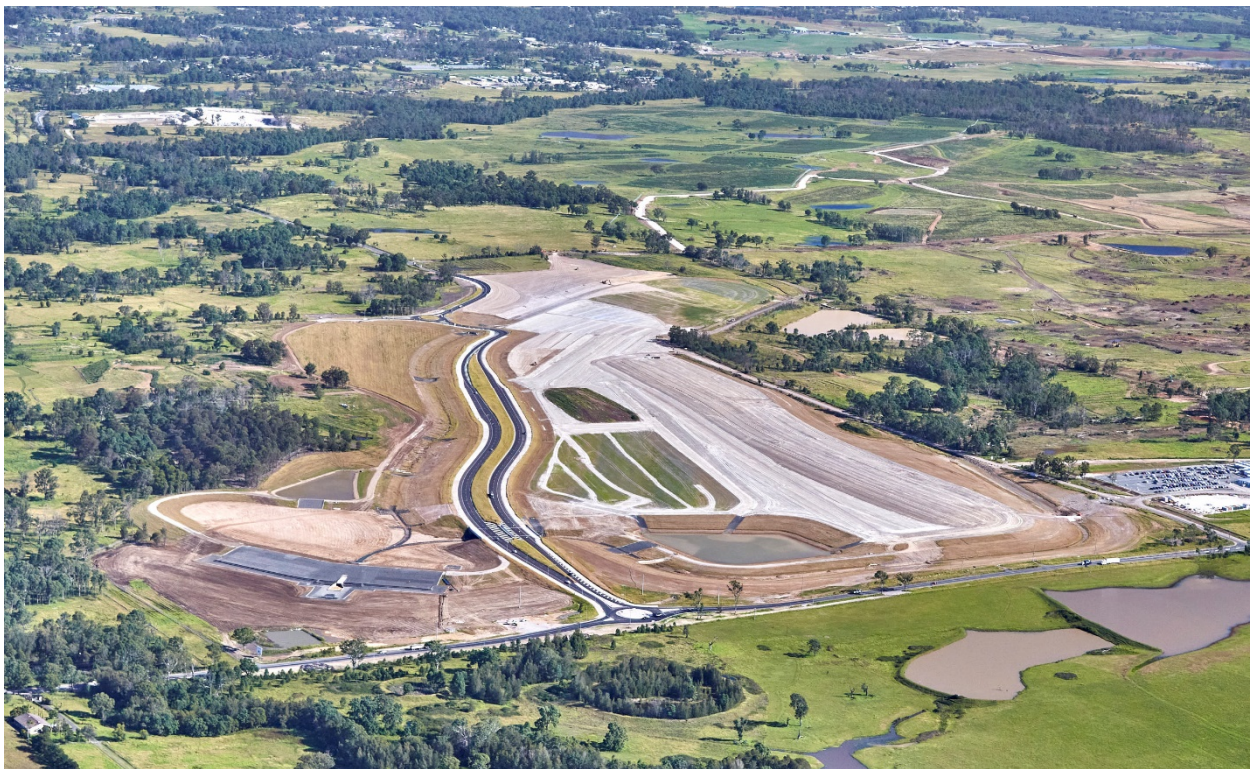
Figure 1: Early Earthworks – April 2020
