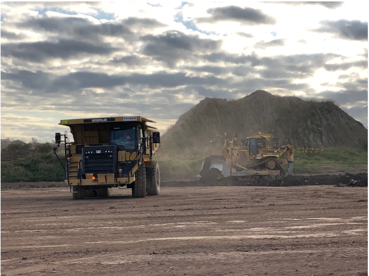
Figure 3: Bulk Earthworks – July 2020
