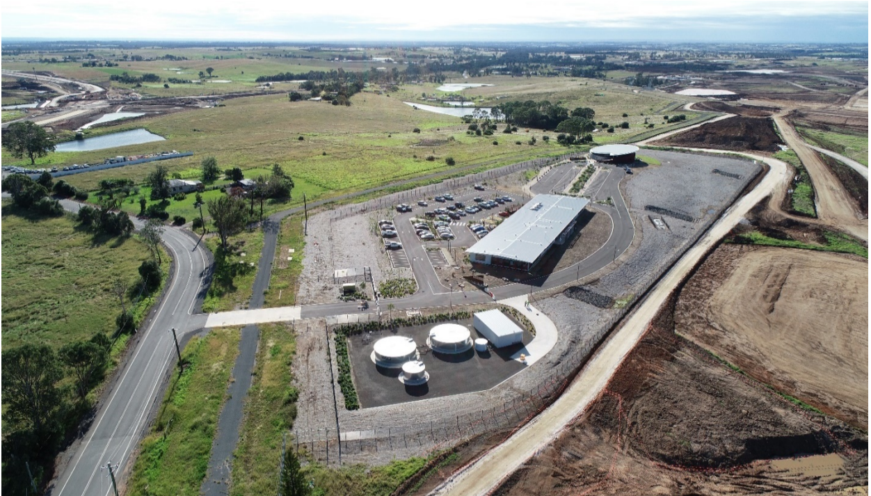
Figure 2: Completed Experience Centre – June 2020
