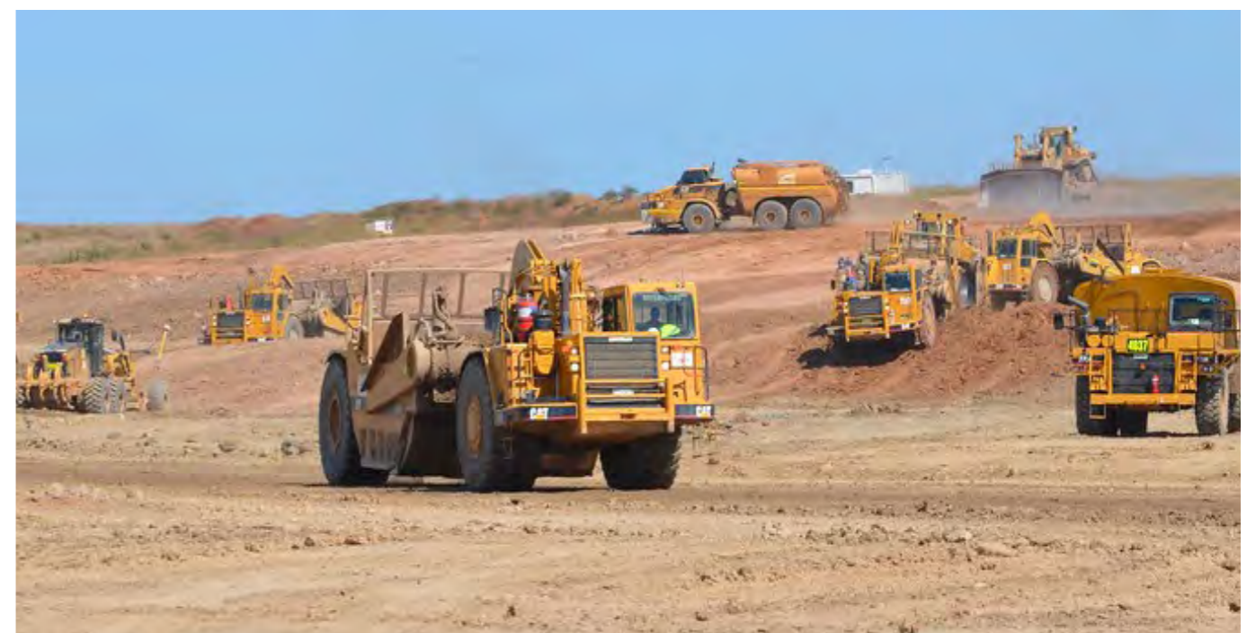
Western Sydney International is one of Australia's largest earthmoving projects.
