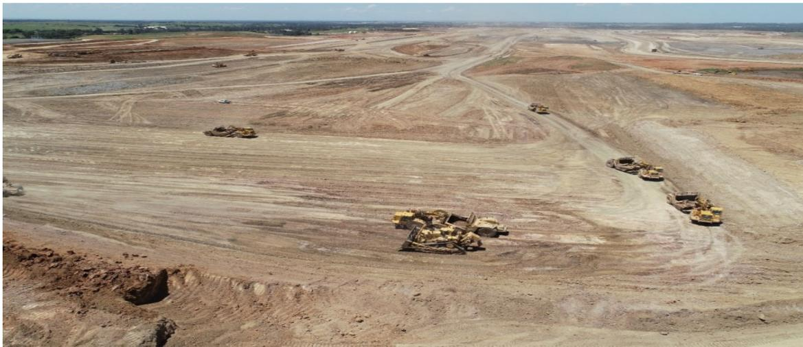
Figure 2: Bulk Earthworks Scrapers and Dozers operating – December 2020
