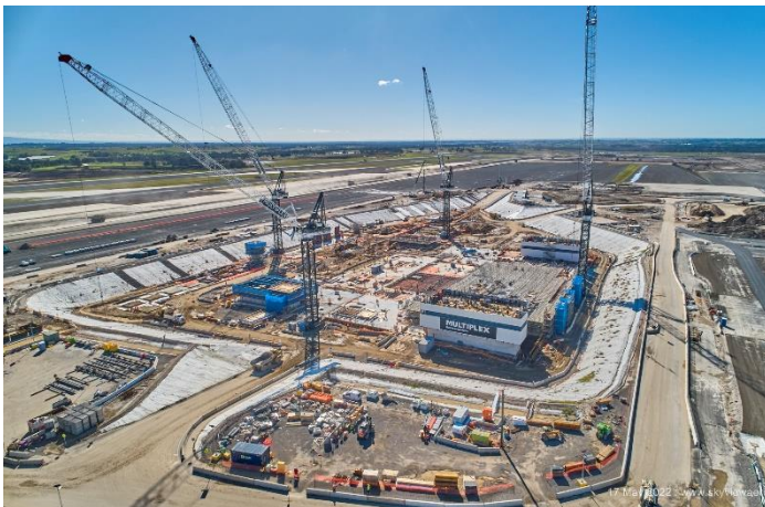
Aerial photo of the terminal basement, taken May 2022
