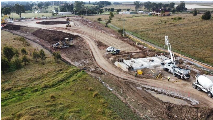
Anton Road looking north, box excavation work and culvert installation underway
