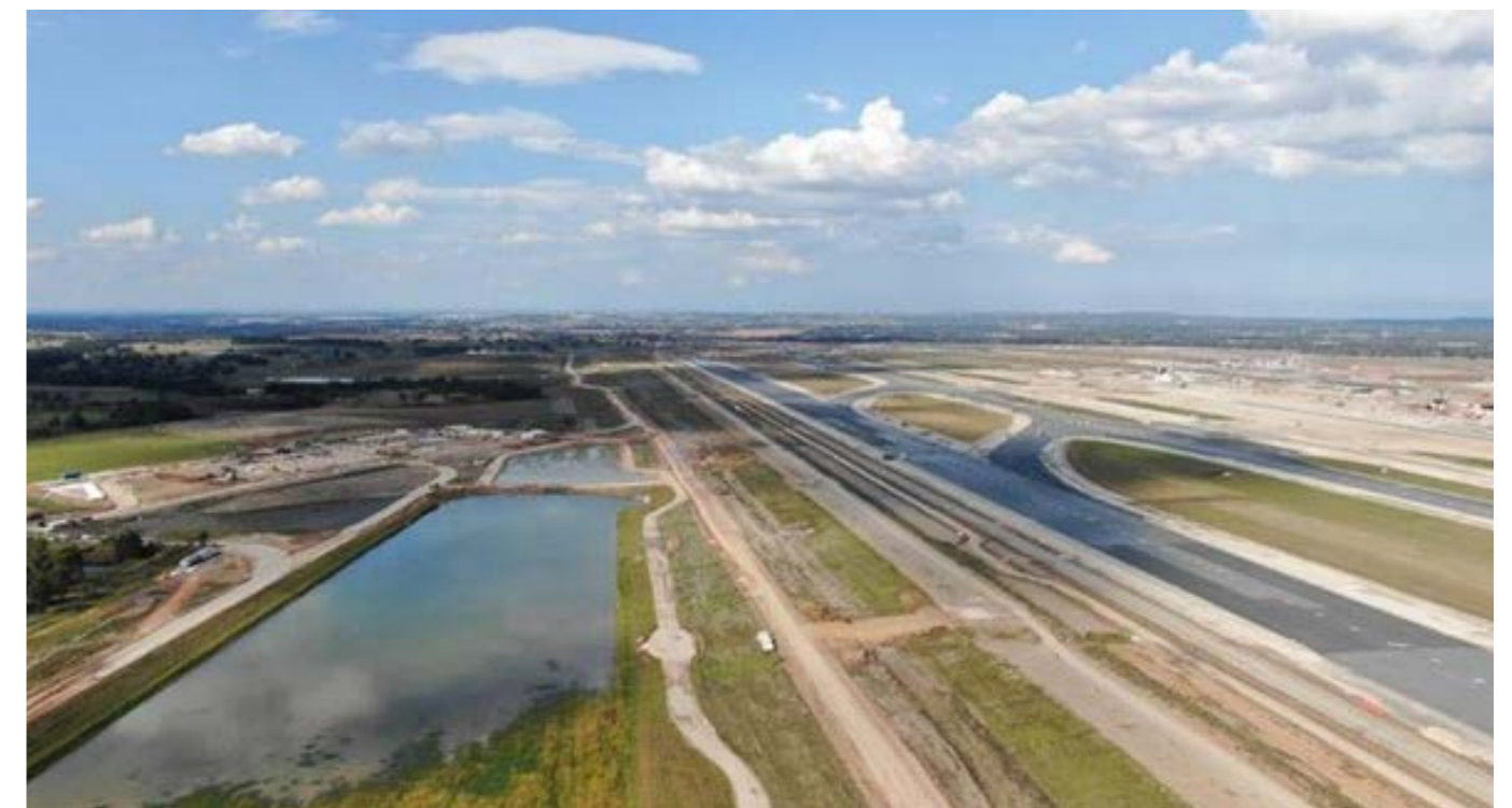
Figure 23 - Basin 7 with water being utilised for dust suppression on site
