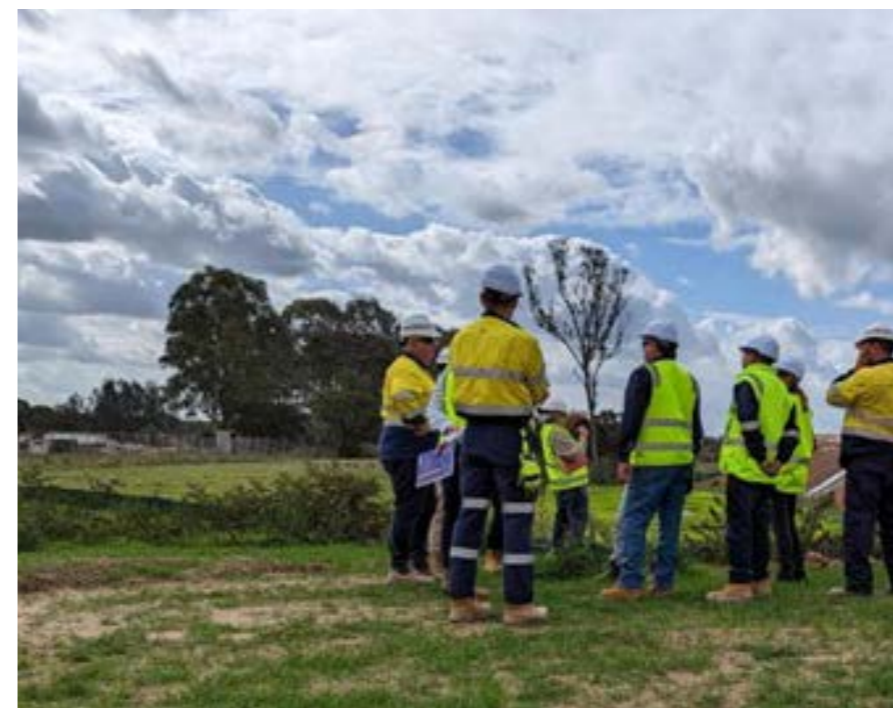
Figure 1 – WSA ERG Undertaking inspection at the Fuel Farm Works with Multiplex
