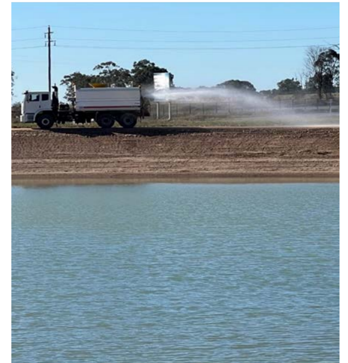
Figure 27 - Reuse of site captured water to reduce dust generation
