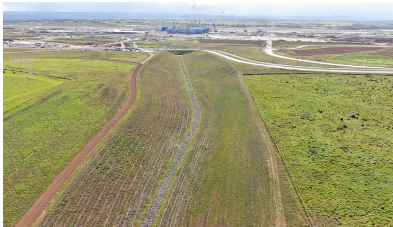
Figure 24 - Grass lined Basin 3 Channel
