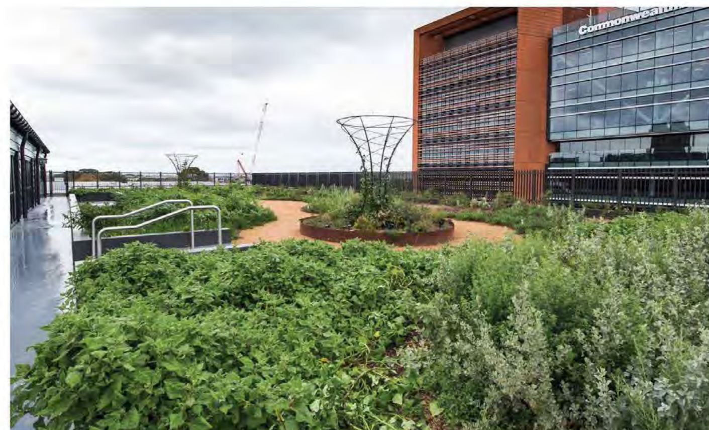
Image showing an example of a communal green roof for a commercial development at Commonwealth Building at Eveleigh, NSW Source: https://www.timeout.com/sydney/attractions/yerrabingin-rooftop-garden
