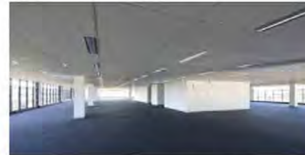
Image: Example precedent at 6 Eden Park Drive, North Ryde Source: Sutton Anderson, Property Consultants
