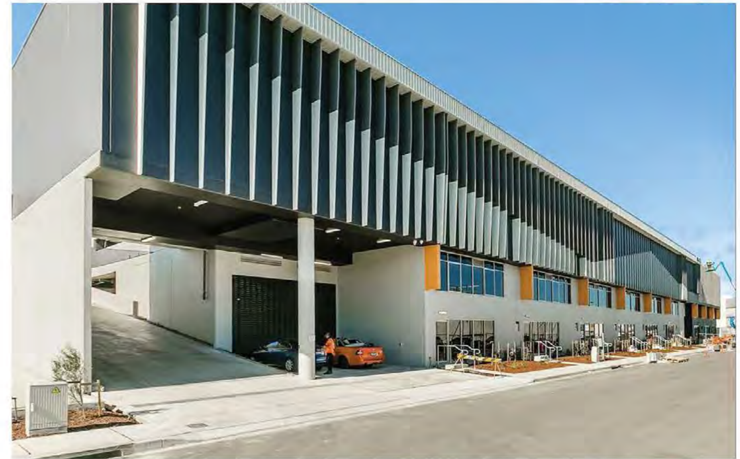
Images above: Example precedents of Enterprise Industrial Estate, 8 Jullian Close Botany Source: https://www.enterpriseindustrial.com.au/
