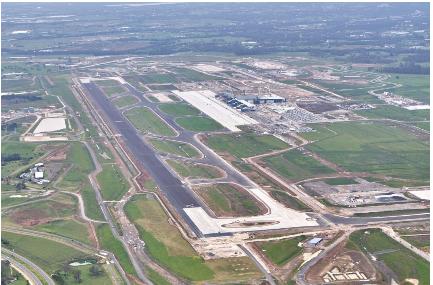
Aerial photo of the site, taken January 2024
