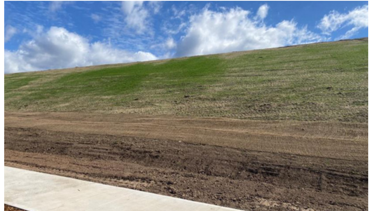
Figure 5 - Flexterra installation on batters to reduce erosion
