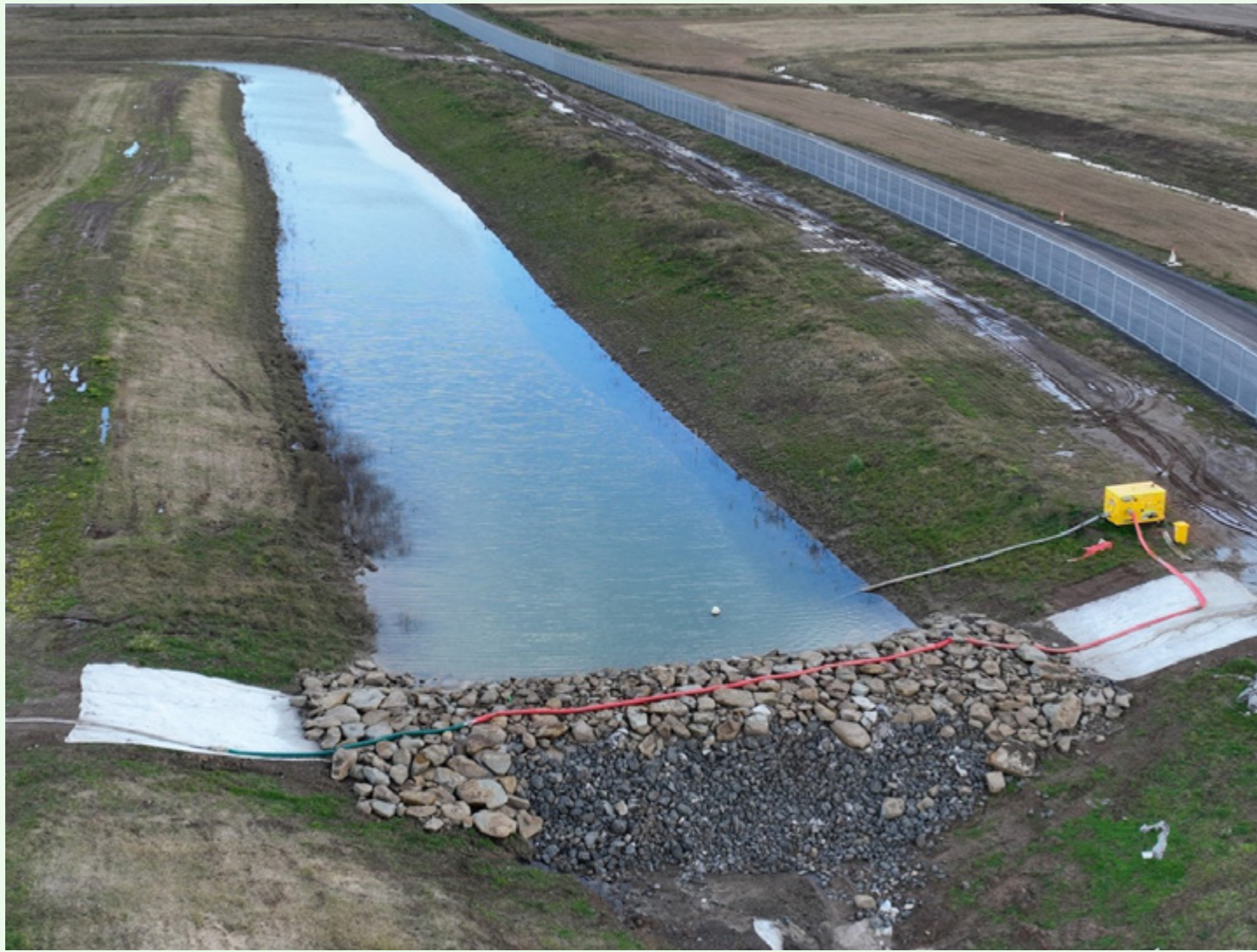
Figure 34 – Cargo temporary basin water being utilised for dust suppression on site
