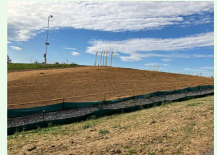
Figure 39 - Rip rap lined channel and the bottom of stabilised batters
