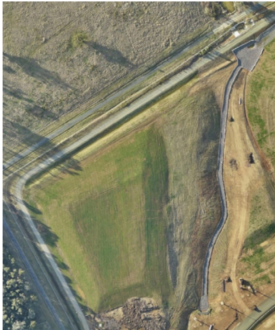
Figure 4 – Rip rap drainage channel in place of grass surface treatment
