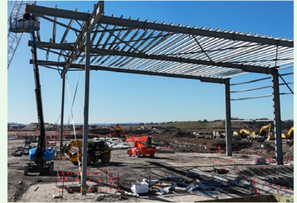
Figure 1 - Initial steel erection on Cargo facility (August 2024)
