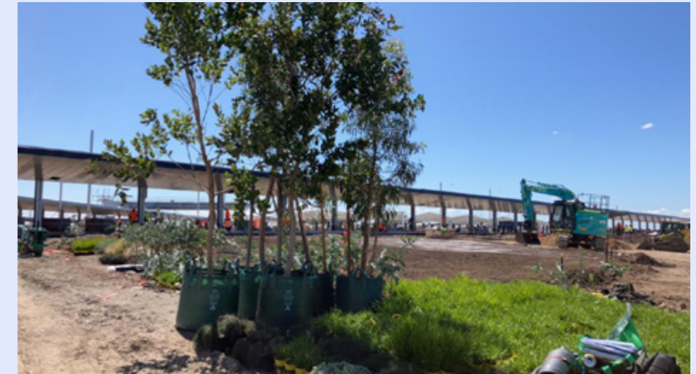
Figure 42 - landscaping works in the Terminal forecourt
