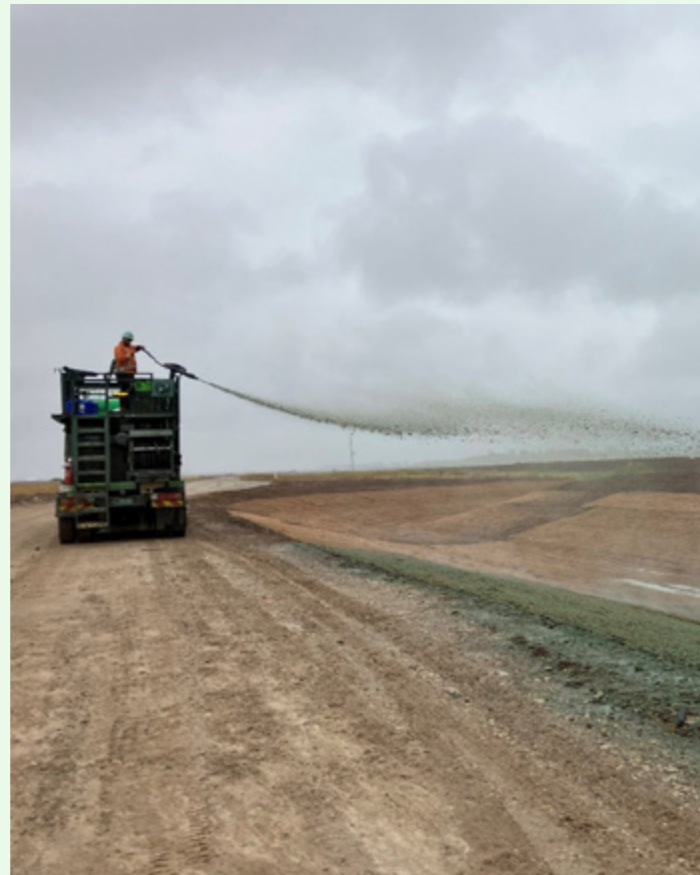
Figure 36 - Hydromulch spraying of open drainage channel
