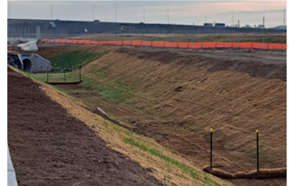
Figure 33 – Jute lined drainage channel
