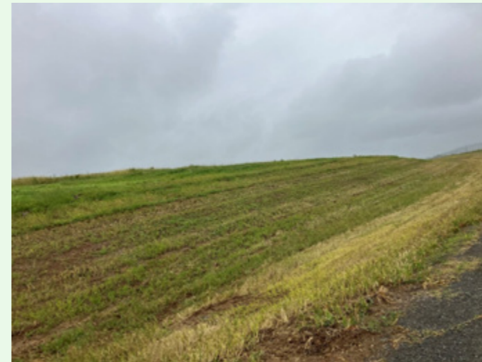
Figure 38 - Grass established on open drainage channel
