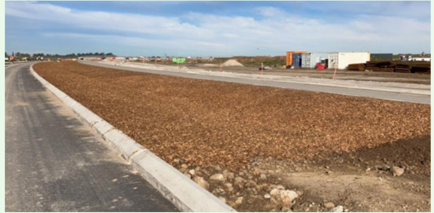
Figure 37 – Mulched swale
