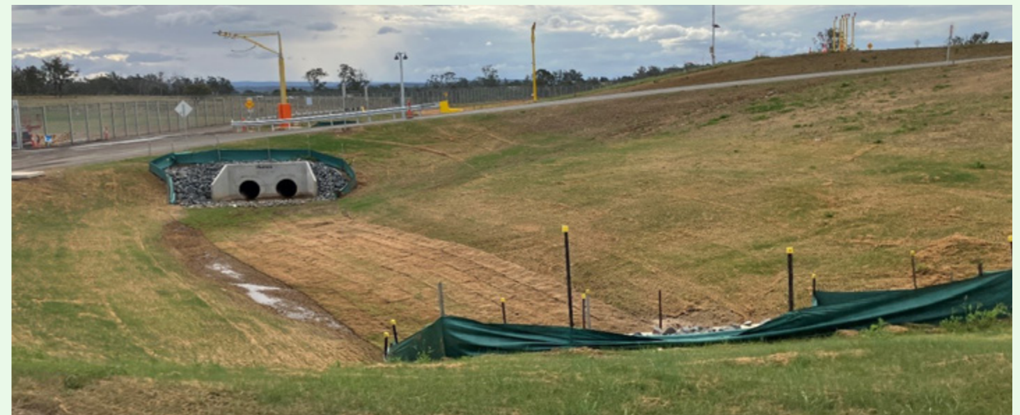
Figure 40 - Turf lined swale
