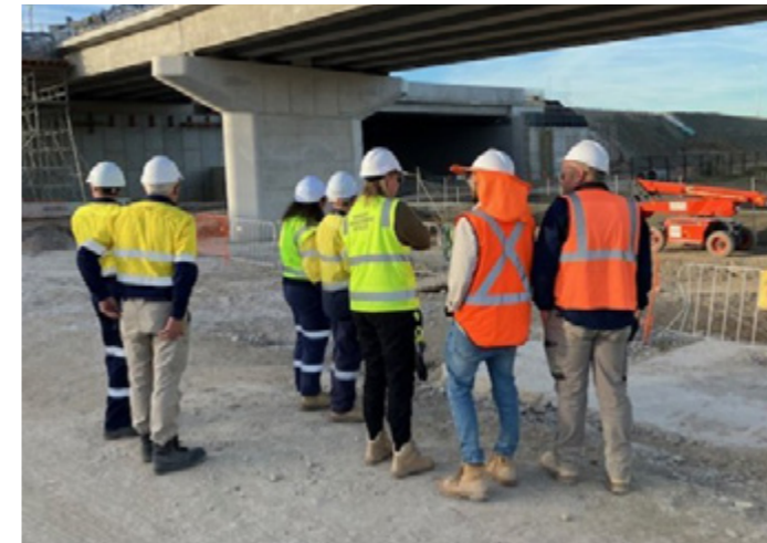
Figure 6 – WSA ERG – AEO undertaking inspection of M12 bridges
