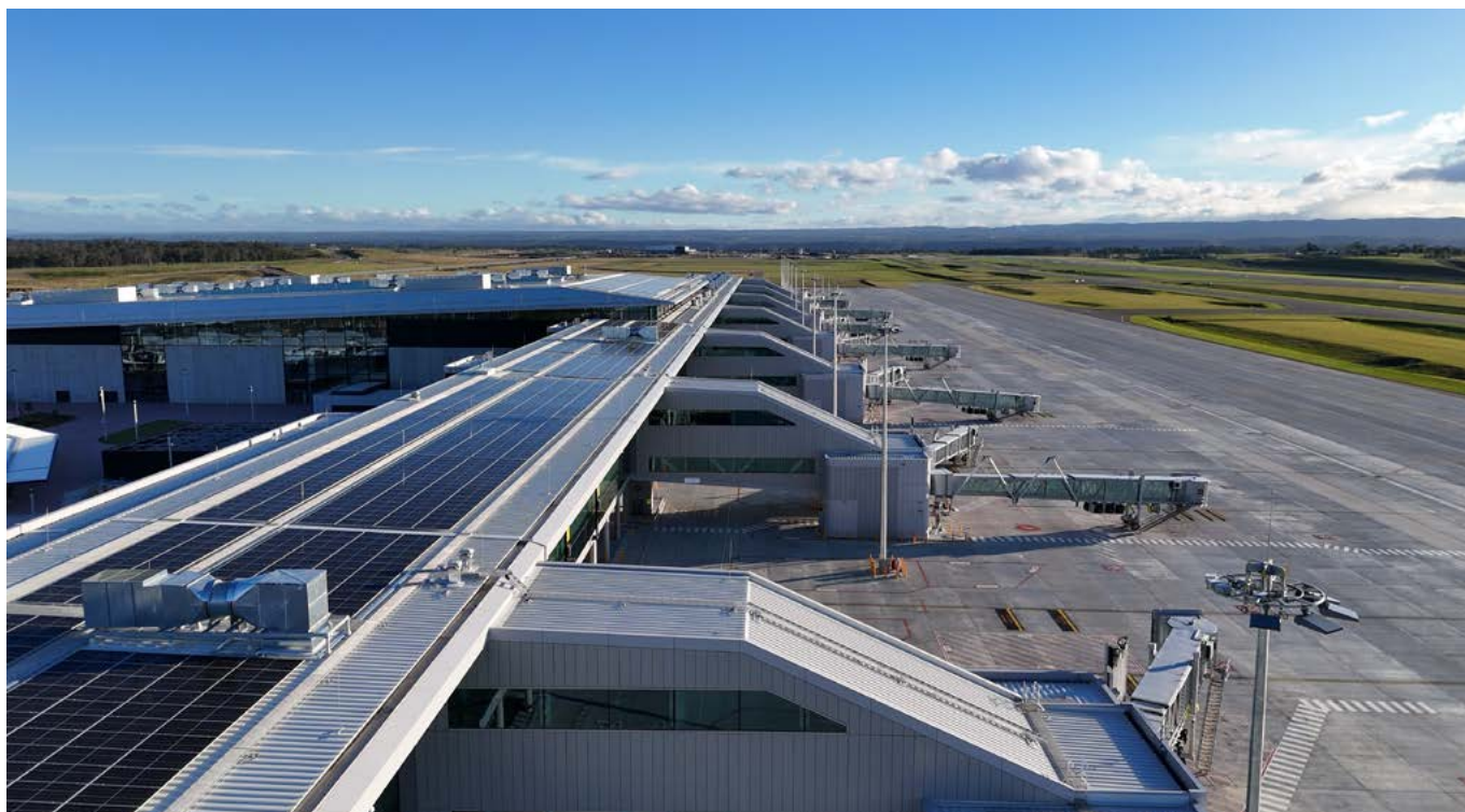
Our terminal roof has over 6,000 solar panels to provide energy efficiency and renewable electricity.
