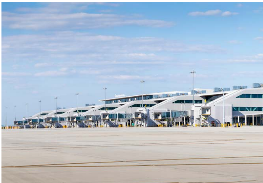
Construction is now complete on our terminal and ready for our 2026 opening.
